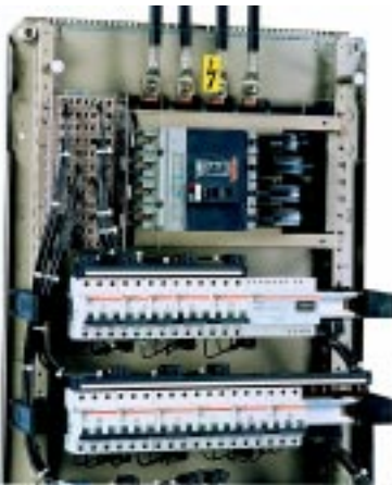
Incoming unit on a 160 A switchboard
